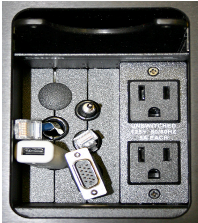
Open Cable Cubby
